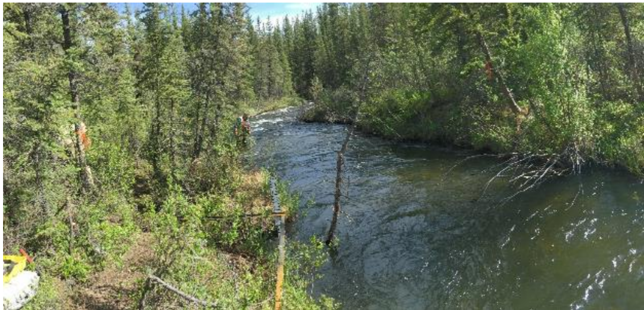
Figure 11 – Fox Creek Hydrometric Station after installation. June 8, 2017
