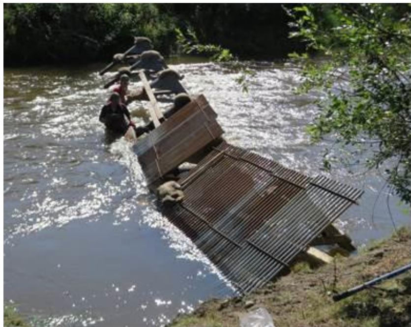
Figure 2. Weir under construction, July 24.
