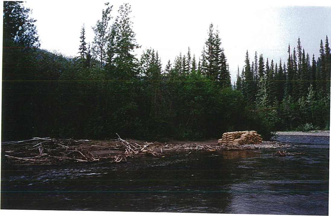
Above: Filling 400 Sandbags for the weir
