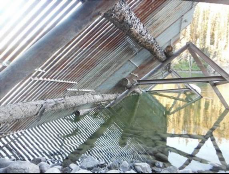
Figure 5. NB diversion weir in place (2013 photo).
