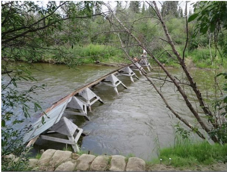
Figure 2. View of fence during construction looking from the west bank.
