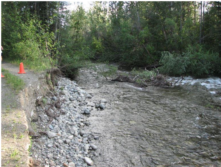
Figure 3. Washout below upper bridge on Blind Creek road due to spring floods.
