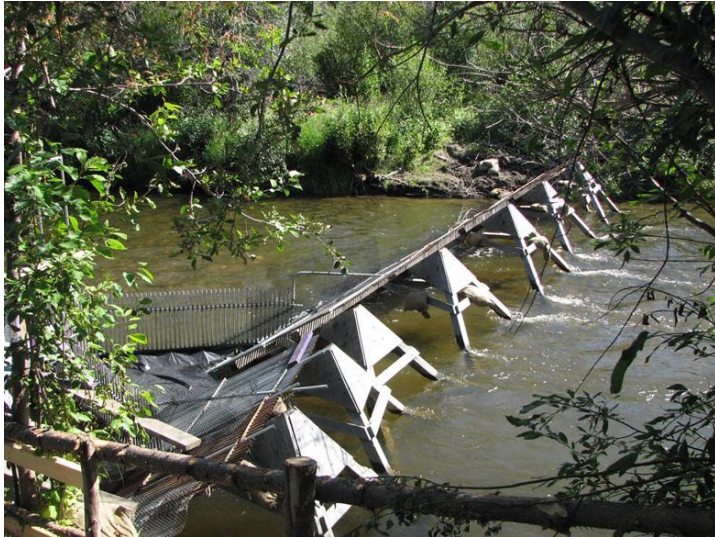
Figure 2. Weir structure looking from west bank.
