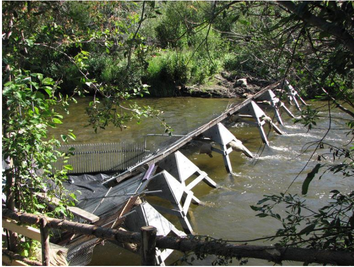
Figure 2. Weir structure looking from west bank.
