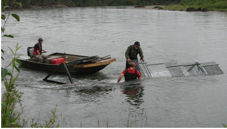
Figure 3. Construction of partial weir on south side of river. (Photo 2011)
