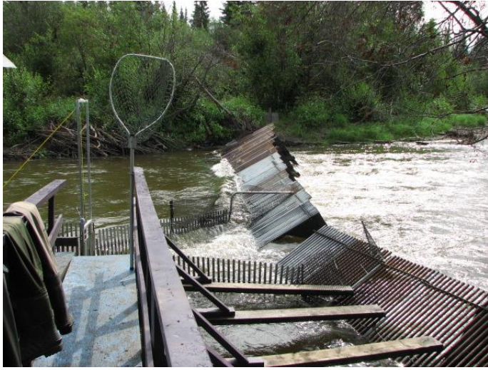
Figure 2. Blind Creek at high water on August 13.
