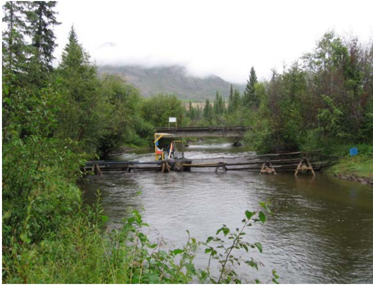
Figure 3. View of weir looking upstream.
