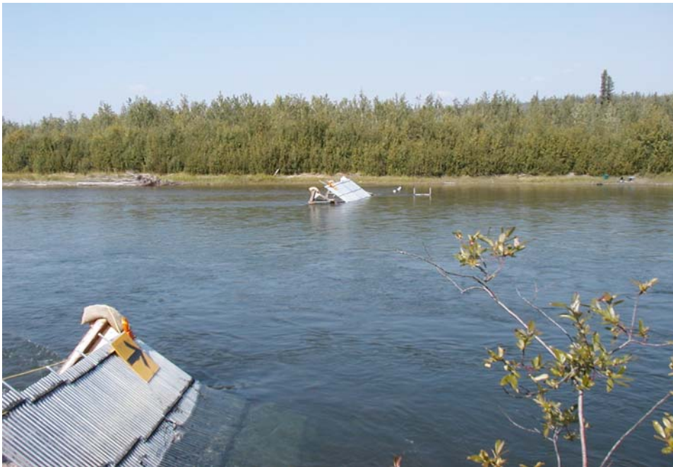
Figure 2. Partial weirs and 34 m opening for fish passage viewed from the south bank.
