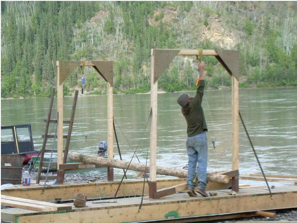
Photo 2. Preparing completed raft for baskets
