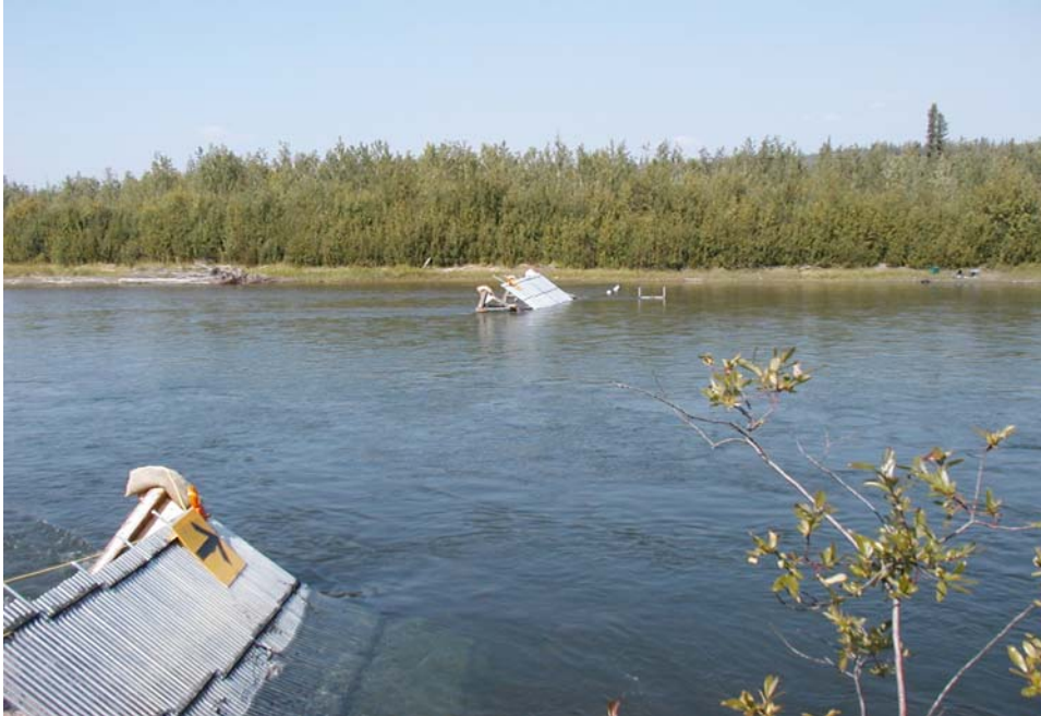
Figure 2. Partial weirs and 34 m opening for fish passage viewed from the south bank.
