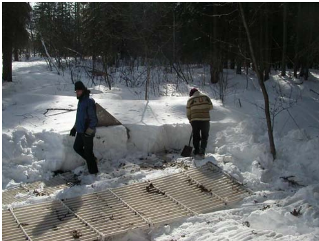
Photo 3: Ron McCready and Jonathon Dowdell digging out weir sections.
