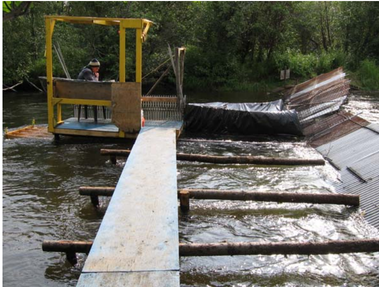
Figure 2. Weir and sampling station viewed from the north bank.
