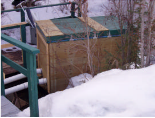
Settling Box: Exterior
