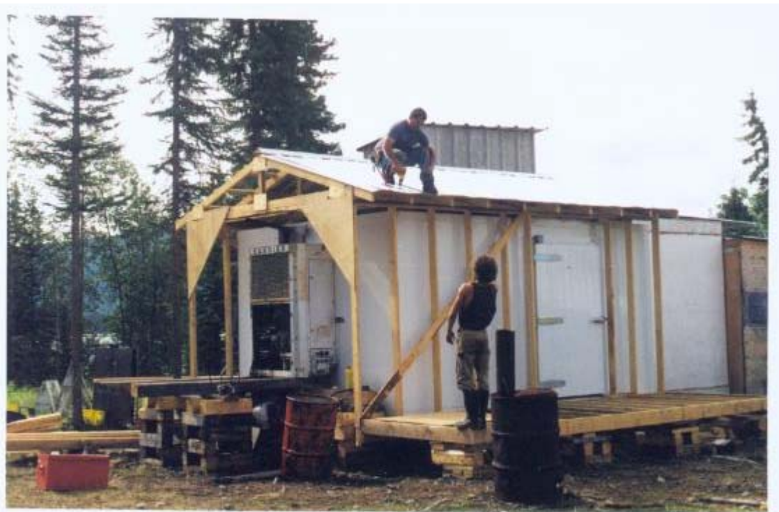
Photo 5. Constructing the enclosure for freezer box on site.
