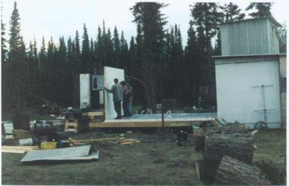
Photo 4. Assembling the freezer box on site.
