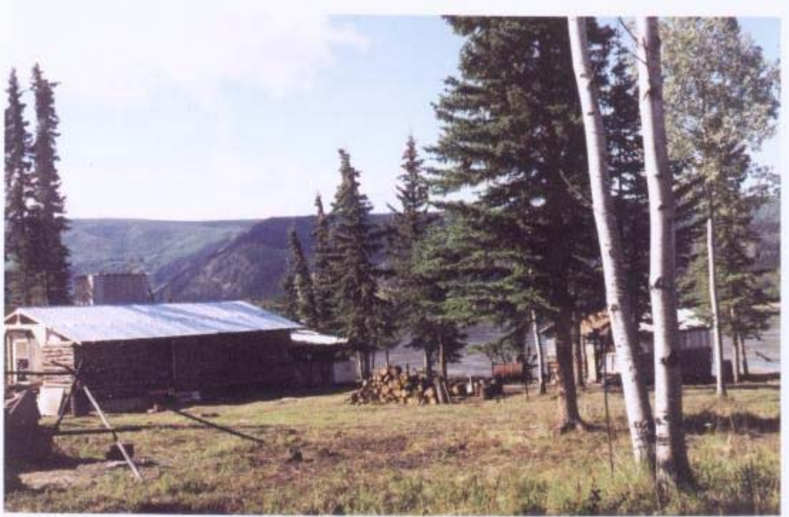
Photo 2. View of Fish Processing Facility with new freezer unit installed.
