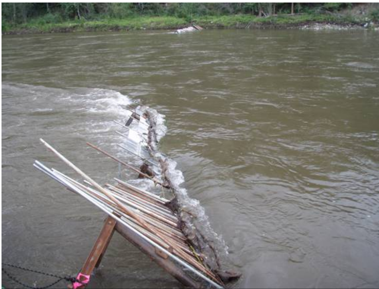
Figure 8. Weir structures in high water conditions, Klondike River sonar site.
