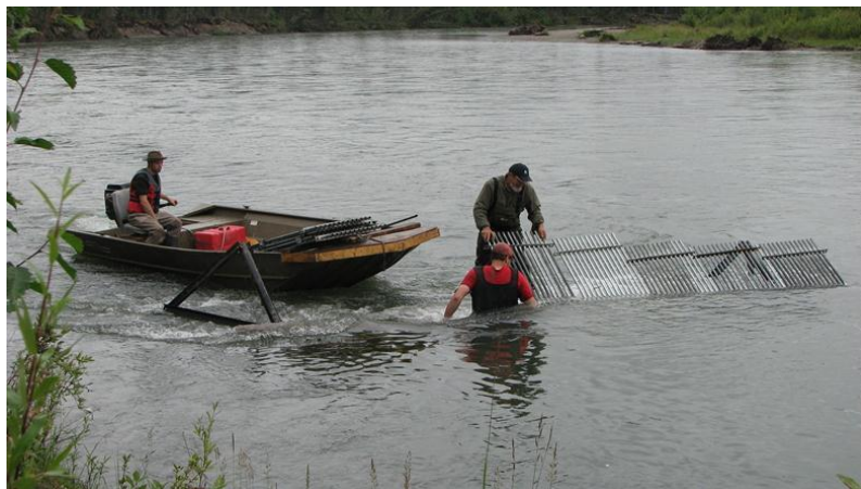
Figure 4. Construction of partial weir on south side of river.
