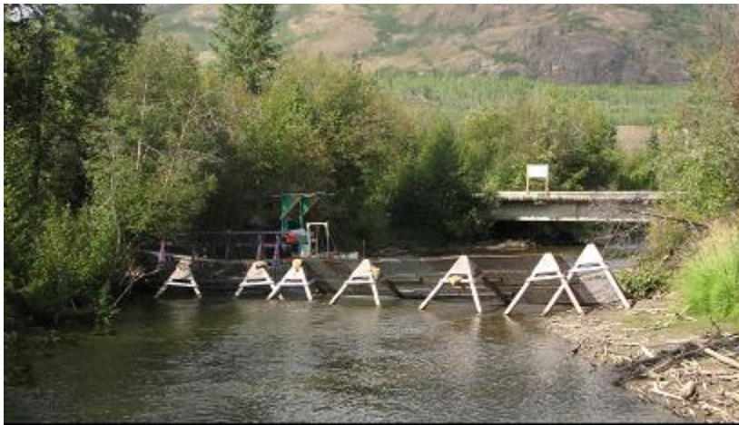
Figure 3. View of weir structure looking upstream.
