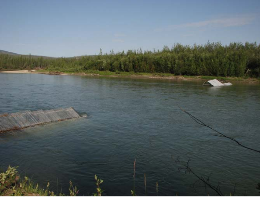
Figure 2. Partial weirs and 36 m opening for fish passage viewed from the south bank.
