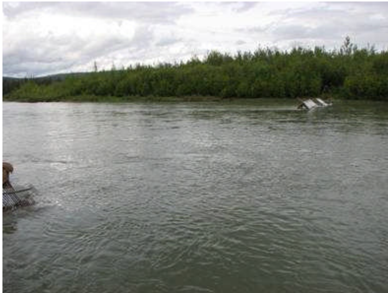
Figure 3. Partial weirs and 34 m opening for fish passage viewed from the south bank.
