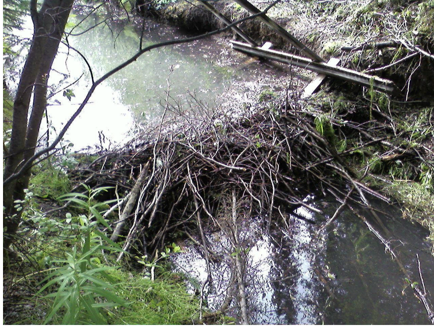
Beaver dam at the downstream screen
